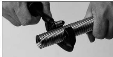
1. Cut hose to required length in the corrugation groove using a pipe cutter.
