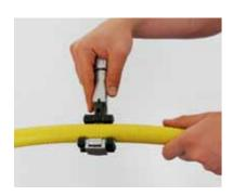
1. After measuring the section to be installed, cut the flexible hose from the reel with a surplus of about 5 - 10 cm.
